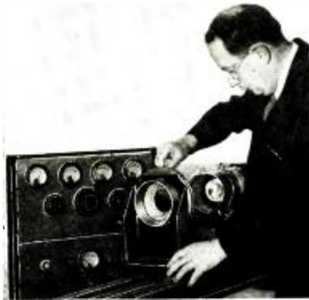
Some of the experimental apparatus employed for wave-guide transmission.
