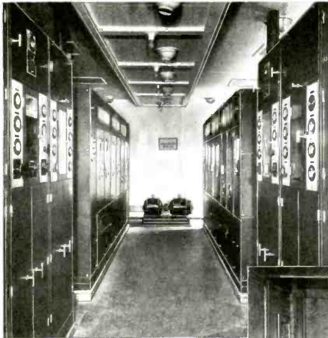
Above—A view of the Radio Transmitter Room of the "Queen Mary." The short-wave transmitters in the foreground, as well as the long-wave transmitters, are operated from a Control Room 400 feet distant.
